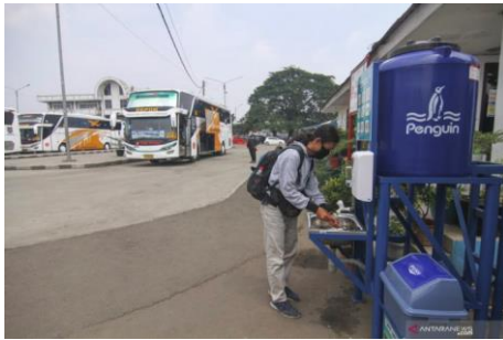
3. Availability of hand wash facility
